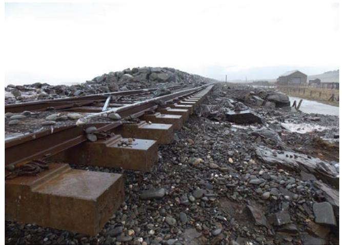
*The impacts of coastal flooding on the railway near Tywyn, Gwynedd. The railway embankment forms part of the coastal flood defence here, as is the case on many coastal railways.*
